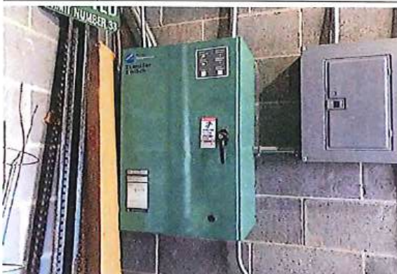
#52 TRANSFER SWITCH, AUTOMATIC (ATS)
