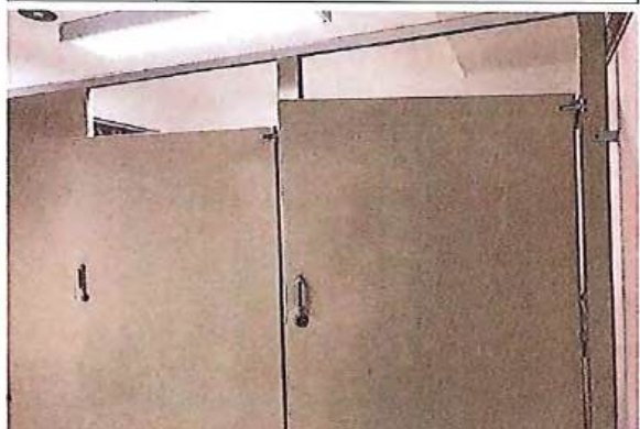
#36 TOILET PARTITIONS, METAL OVERHEAD-BRACED
