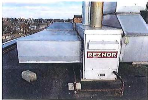
#44 RTU, GAS FOR HEAT RECOVERY SYSTEM
