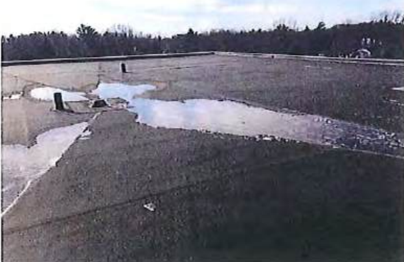
#17 ROOF, SINGLE-PLY EPDM MEMBRANE
