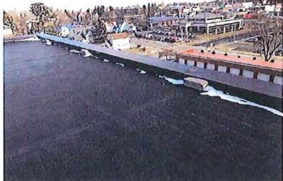
#18 ROOF, SINGLE-PLY EPDM MEMBRANE
