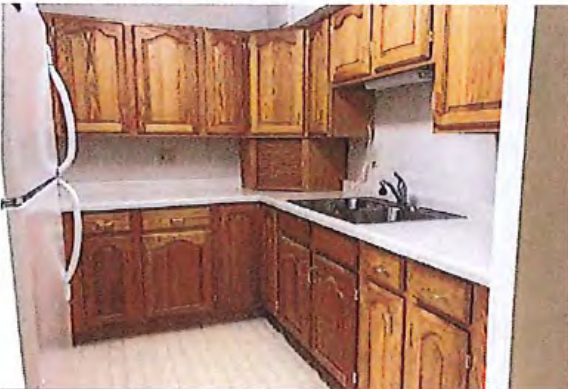
#69 KITCHEN CABINET, BASE AND WALL SECTION, WOOD, REPLACE
